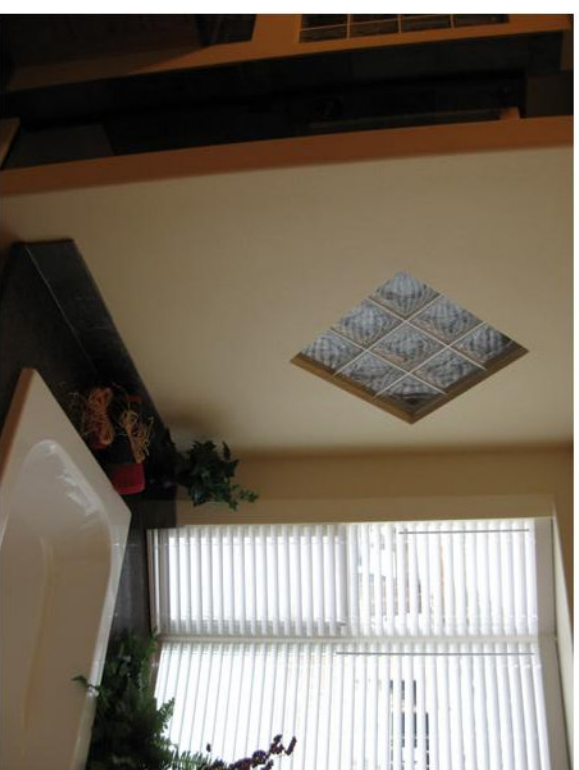
Decorative glass blocks in shower stall adding natural light into shower and a touch of elegance to the appearance of the bathroom
